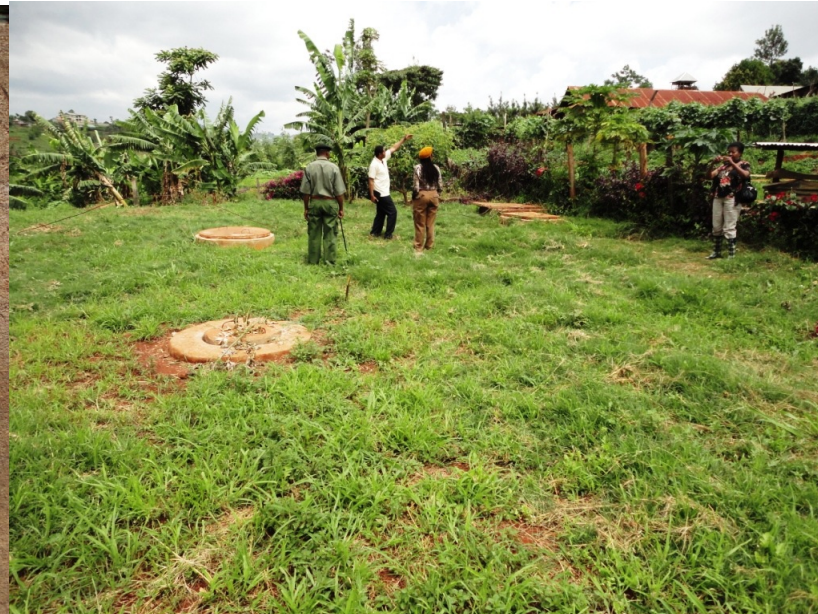
biogas digester completely underground and clean
