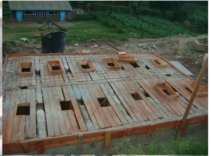
CASTING THE TOP SLAB OF THE BAFFLE REACTORS
